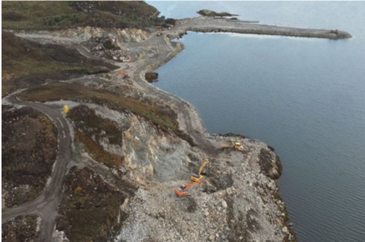
Blasting and movement of rock will continue in October
