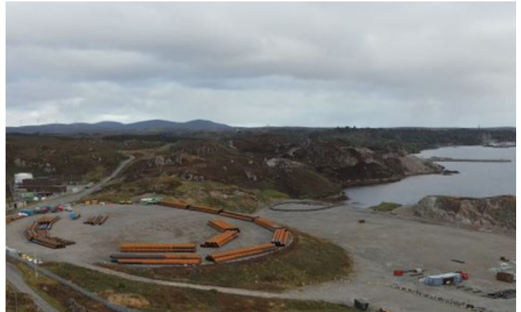
Materials for the quay walls in the site storage compound
